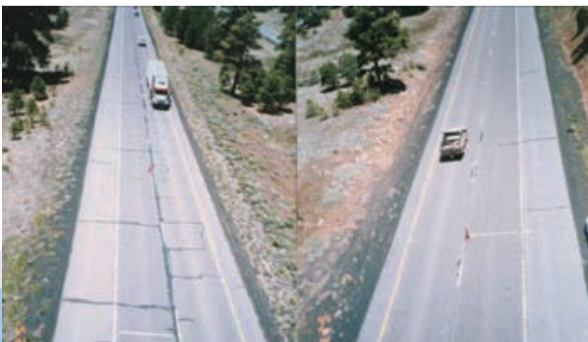
Picture (left): After 8 years the improved quality of CR Modified Asphalt becomes visible. The left side of the picture shows regular asphalt, while the right side shows CRM Asphalt.
